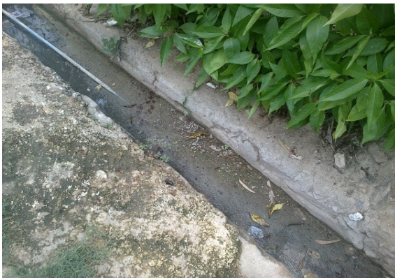
Drainage in Devgiri village of Haveri Taluk (water logging due to improper slope)
