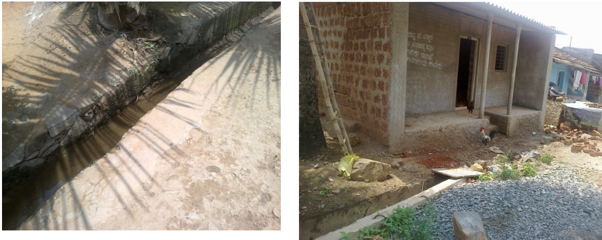
Drainage in Vannahali village of Shiggoan Taluk
