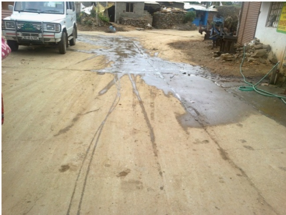
Road in Devgiri village of Haveri Taluk(Left- Water flowing on the Road, Right – Improper levels and Mud accumulated on the Road)
