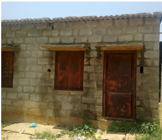
Anganwadi in Manchanabele Village of Chikkaballapura Taluk walls raised on Drainage as foundation
