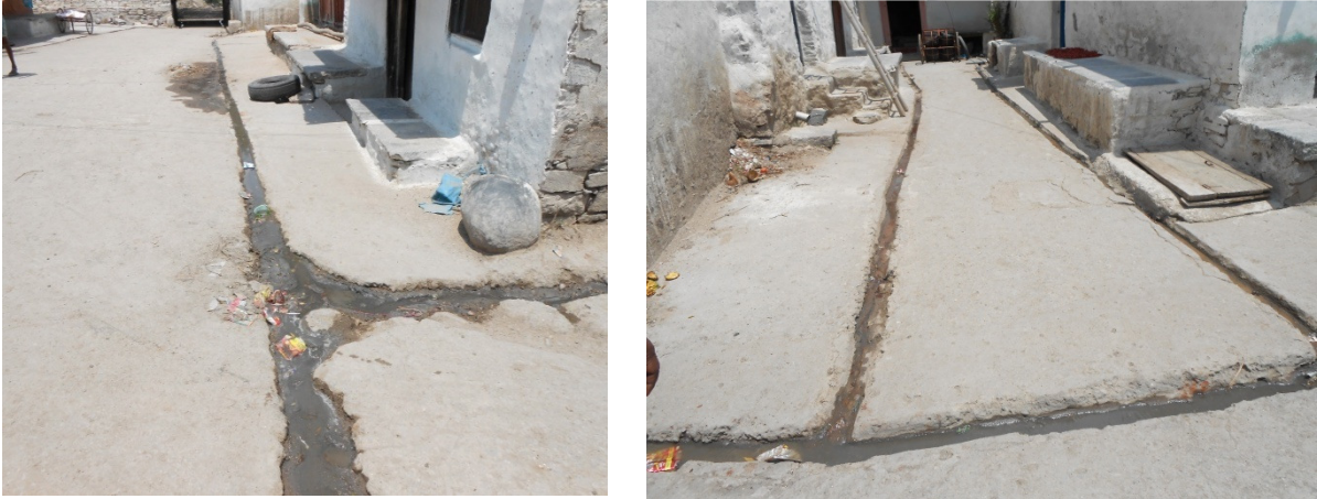
Drainage in Hallikeri village of Gadag Taluk
