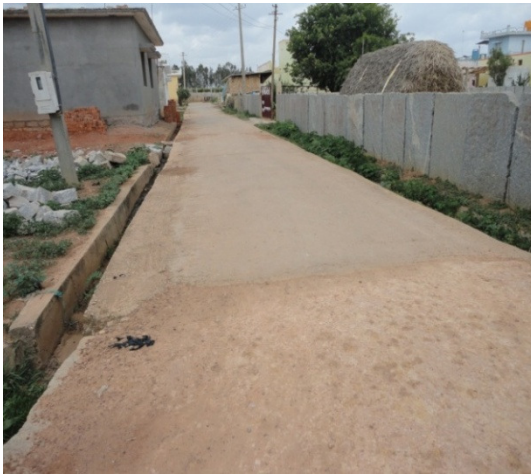
Road in Channarayapattana Village of Devenhalli Taluk( Road with Side Drains)
