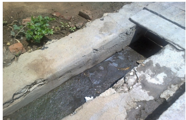
Drainage in Devgiri village of Haveri Taluk (water logging due to improper slope)
